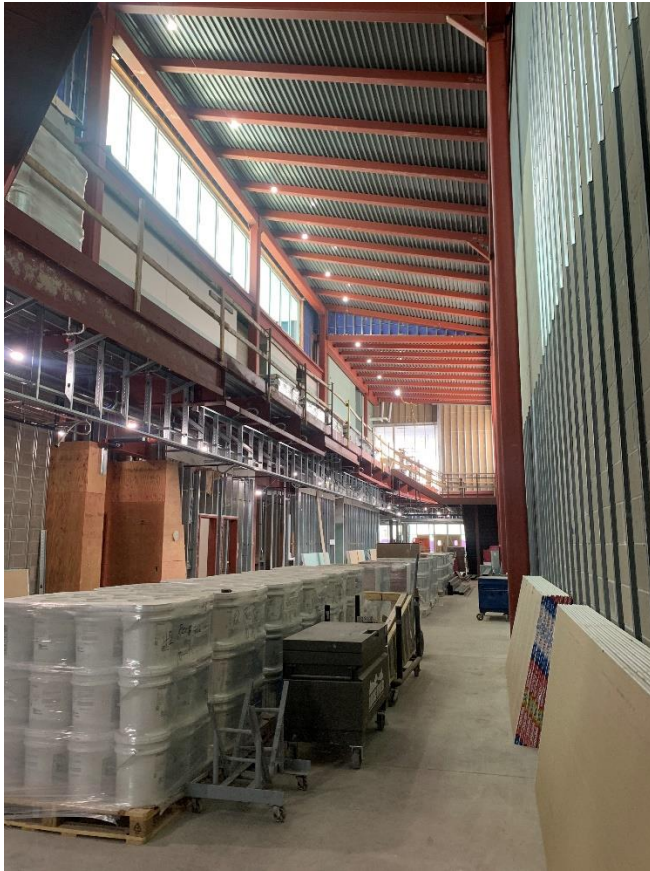
37. Area 1A – Gyp board and metal stud furring strip install at LMC entry in progress.
