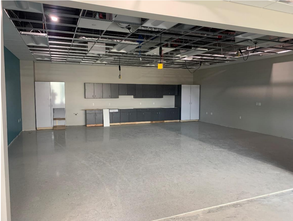
18. Area 6 – Second floor gradewalling entry corridor ceiling grid installed. Electrical fixture install in progress.
