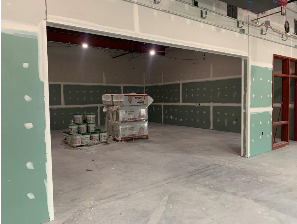
31. Area 4 – First floor gyp board taping and mudding in progress.
