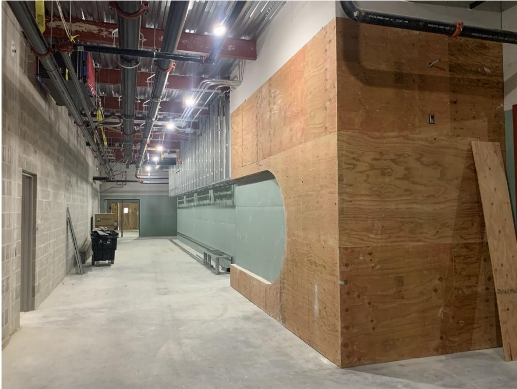
27. Area 3 – Plywood backing, gyp board, and metal stud framing in gradewing entry corridor in progress.
