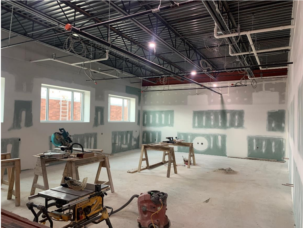
24. Area 3 – Gyp board taping, mudding, and ceiling soffit continues in second floor flex café.
