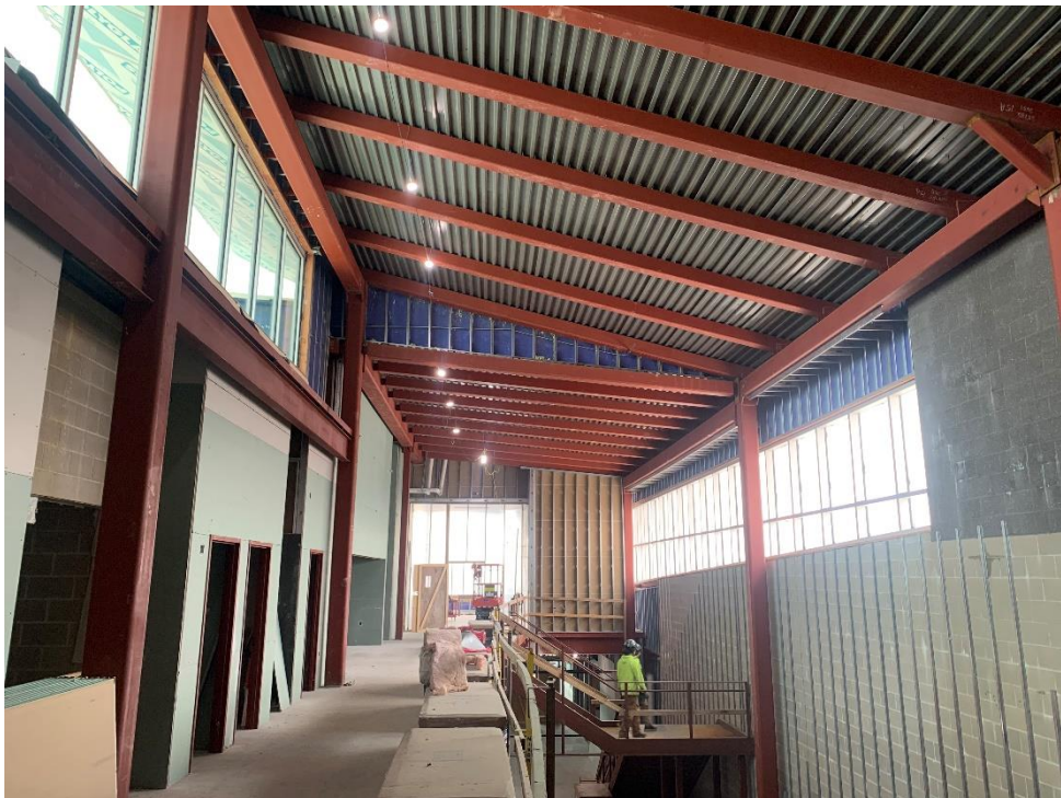
37. Area 1A – Gyp board and metal stud furring strip install at LMC entry in progress.
