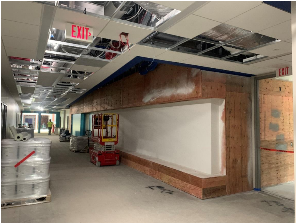
19. Area 5 – Second floor locker pads installed.
