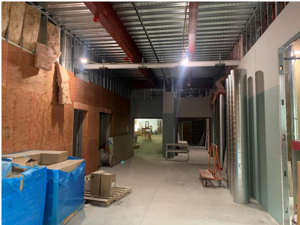
36. Area 1A – Gyp board and plywood backing install continues in gym entry corridor.
