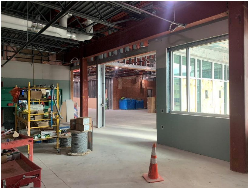
35. Area 1A &1B – Gyp board install in school offices near completion.
