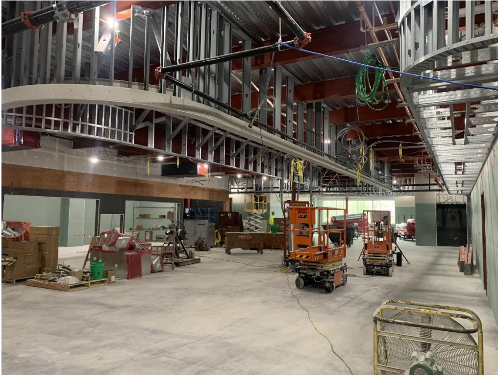
29. Area 3 – Heat pump, above ceiling MEP, and ceiling soffit install in progress.
