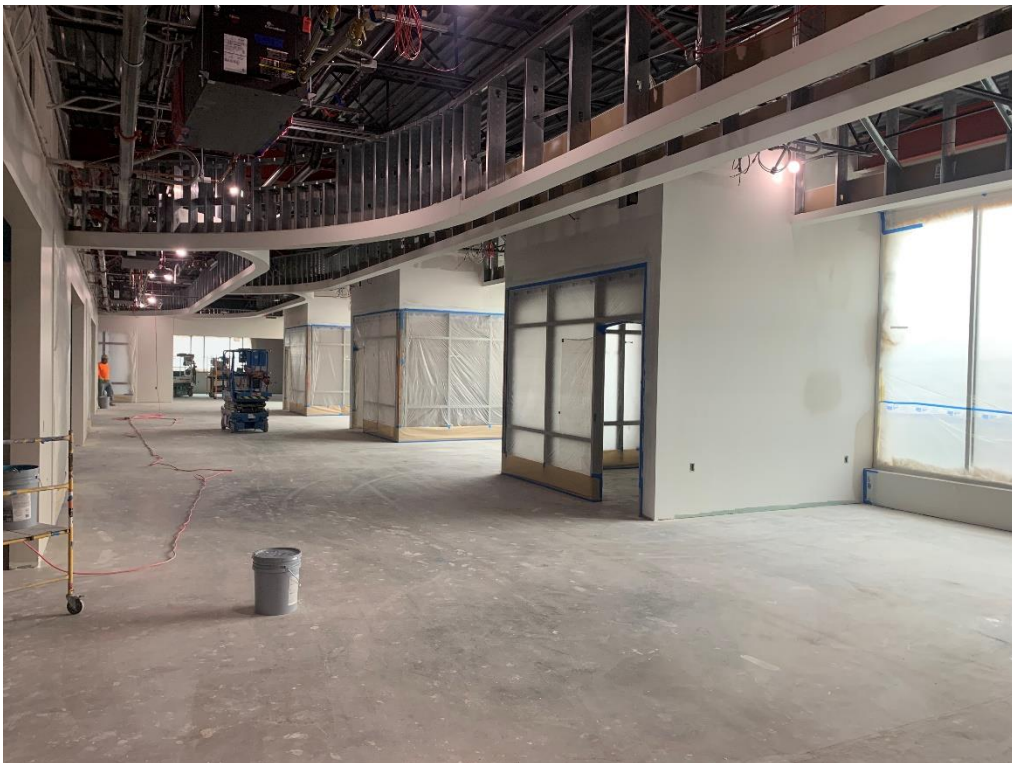
26. Area 4 – Collab area ceiling soffits are installed.
