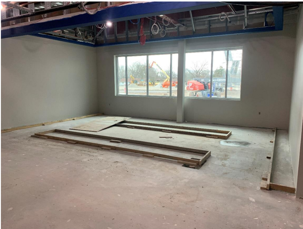
13. Area 5 – First floor classroom glass sliding doors, interior storefront glazing, and casework install are in progress.
